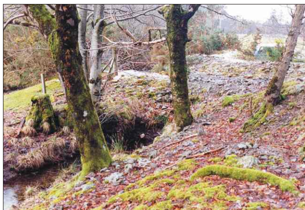
Allt Glac Odhar 'aquaduct' over Foich roadside ditch. During dry periods, most of the water in the Glac Odhar burn percolates through the stream bed into the Foich ditch (P Cunningham)
