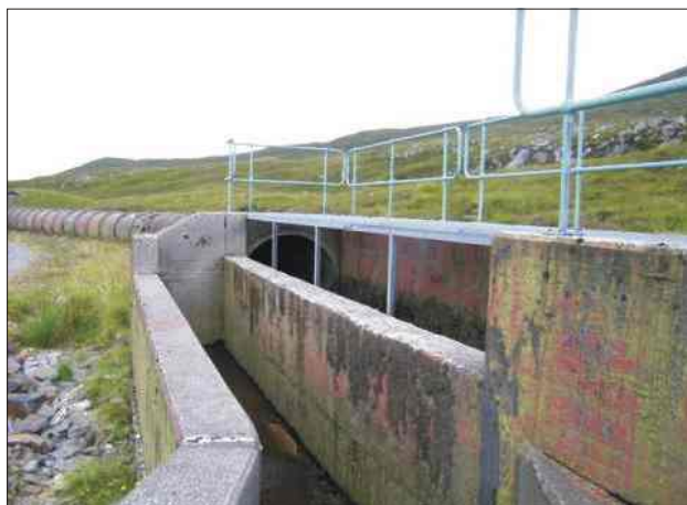
Pipeline diverting water from Allt a' Mhadaidh to Loch Droma. Much of the water from a substantial part of the Droma catchment is directed to Loch Glascarnoch (P Cunningham)
