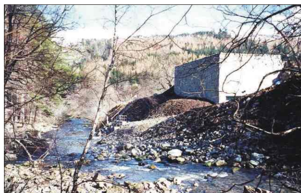
Cuileig Power station. Loose sediment from below the power house was washed downstream into the Junction pool (P Cunningham, February 2002)
